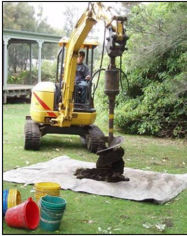
Excavating a mechanical auger test pit
