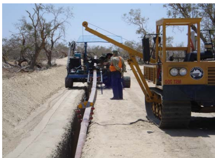
Plate 4.3 Gas Flow Line Placement
