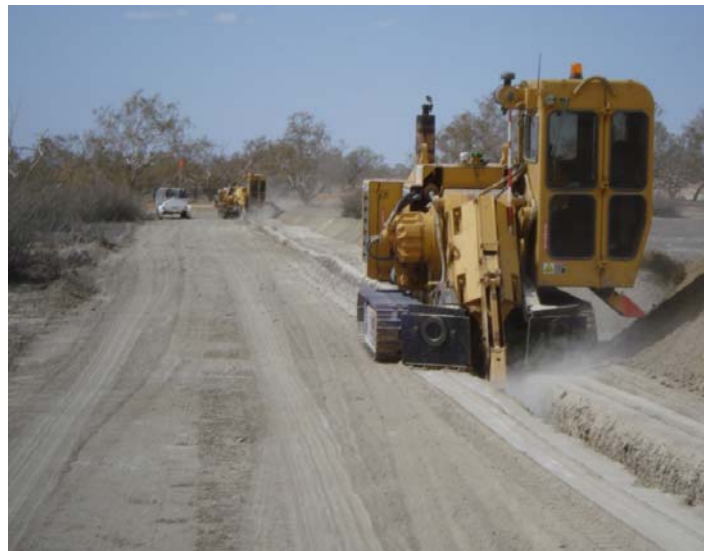
Plate 4.1 Trenching Process
