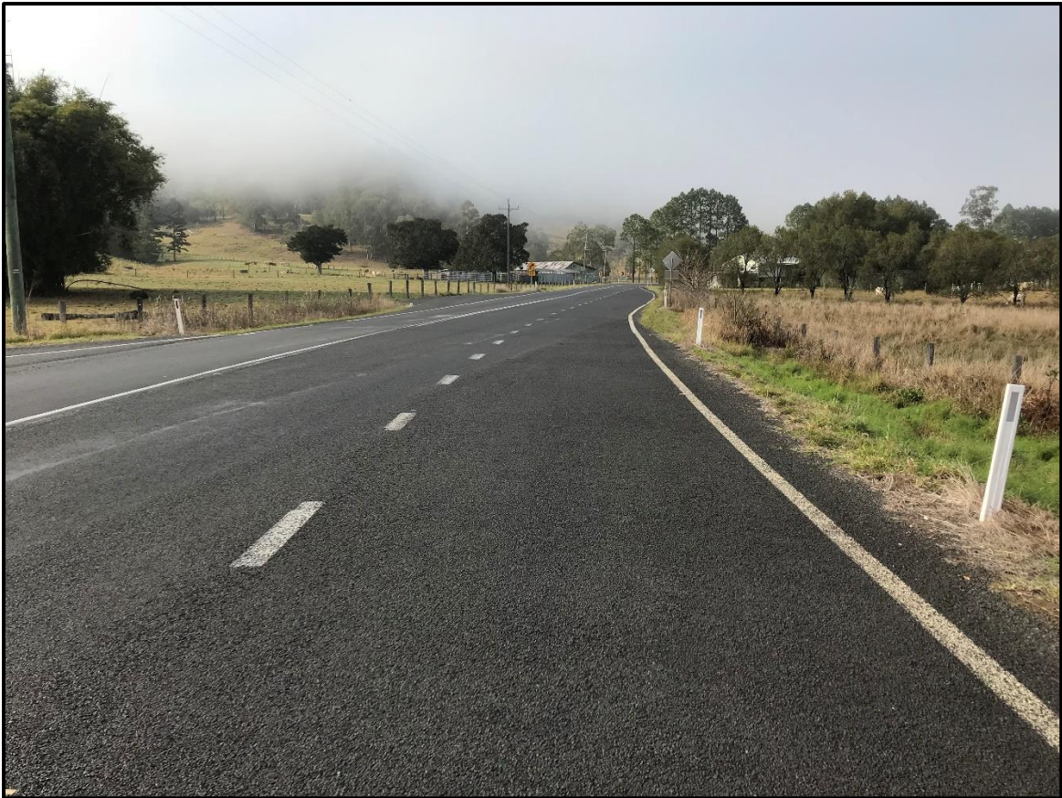
Photo 3 – AUR provided on Nimbin Road for the right turn movement into the Quarry Access Road
