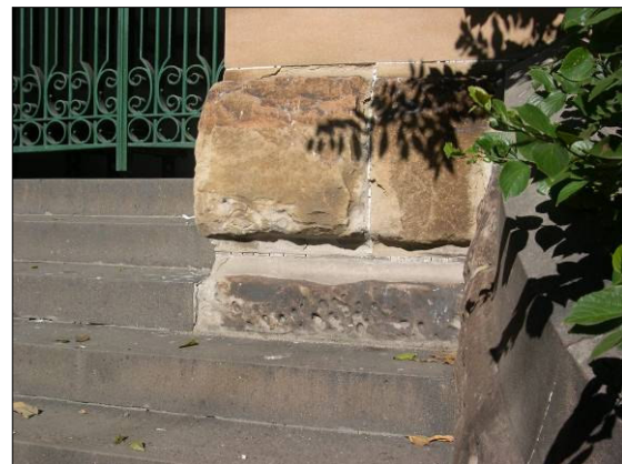
Figure 3: Main arched entrance and the central portico of the Court House (left); the fretting and deterioration of the stone fabric is clearly evident on the main façade (above).
