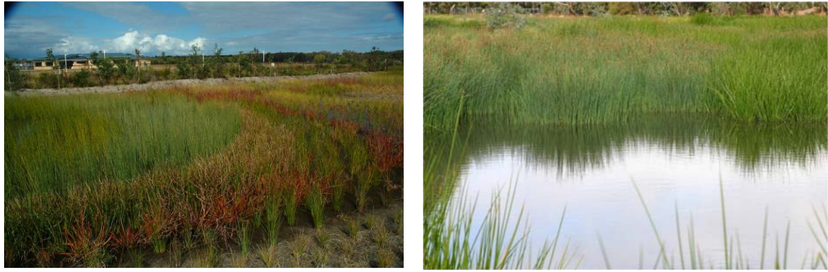
Figure 8 Constructed wetland showing densely planted vegetation in bands shortly after establishment (left) and after establishment, adjoining open water (right). Dense planting promotes efficient water filtration, and resists erosion and weed infestation (design and construction supervision by AECOM).
