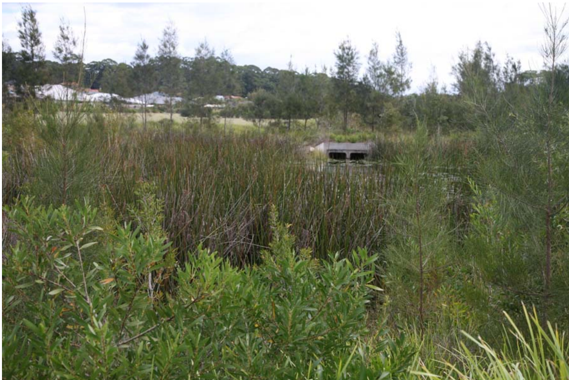
Figure 19 Existing constructed wetland for stormwater treatment at Rainbow Beach. Note the dense growth of aquatic macrophytes in the foreground, with open water and the discharge outlet in the background (Photo taken June 2010).
