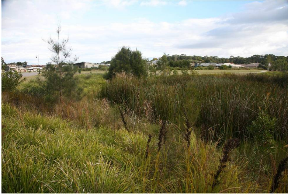
Figure 13 Existing constructed wetland for stormwater treatment at Rainbow Beach Estate. Note the dense edge planting that deters ingress towards the water.
