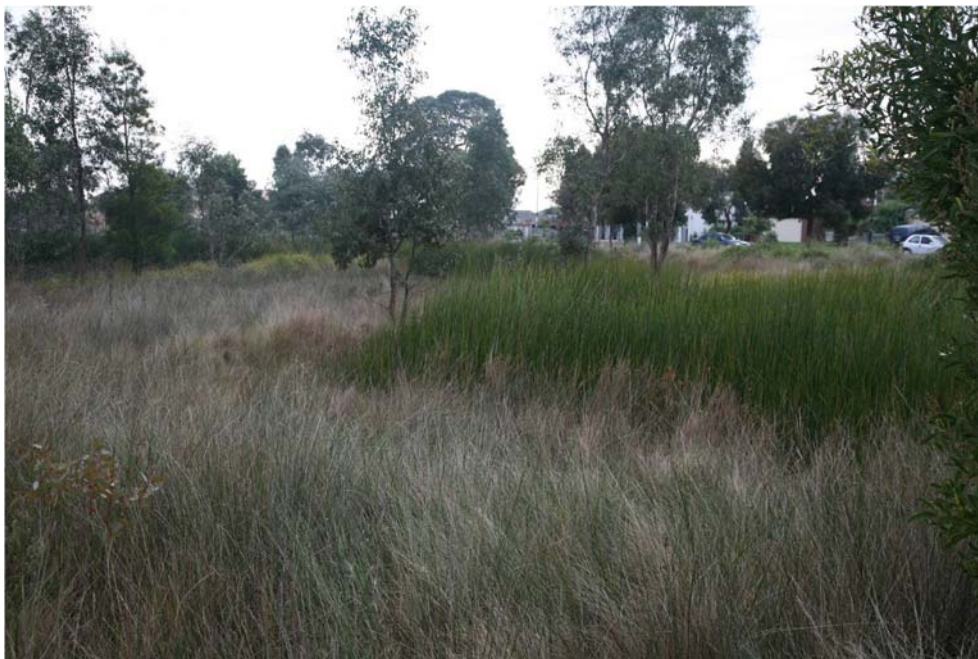
Figure 14 Dense macrophyte planting within a constructed wetland for stormwater treatment. 10 years after establishment the wetland is very resistant to weed invasion (AECOM project, Lynbrook Estate, Victoria).
