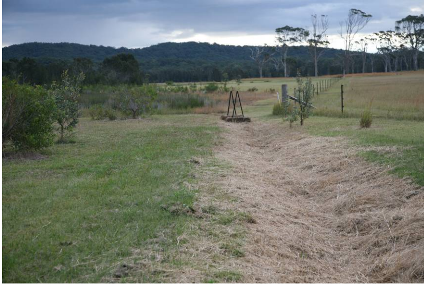
Figure 6 The surface drain that controls inundation depth and runoff from the Marshland (looking upstream). Note the Marshland in the background. Hay bales have been placed in the drain to compensate for the flow control that would have been provided by the grass prior to slashing.
