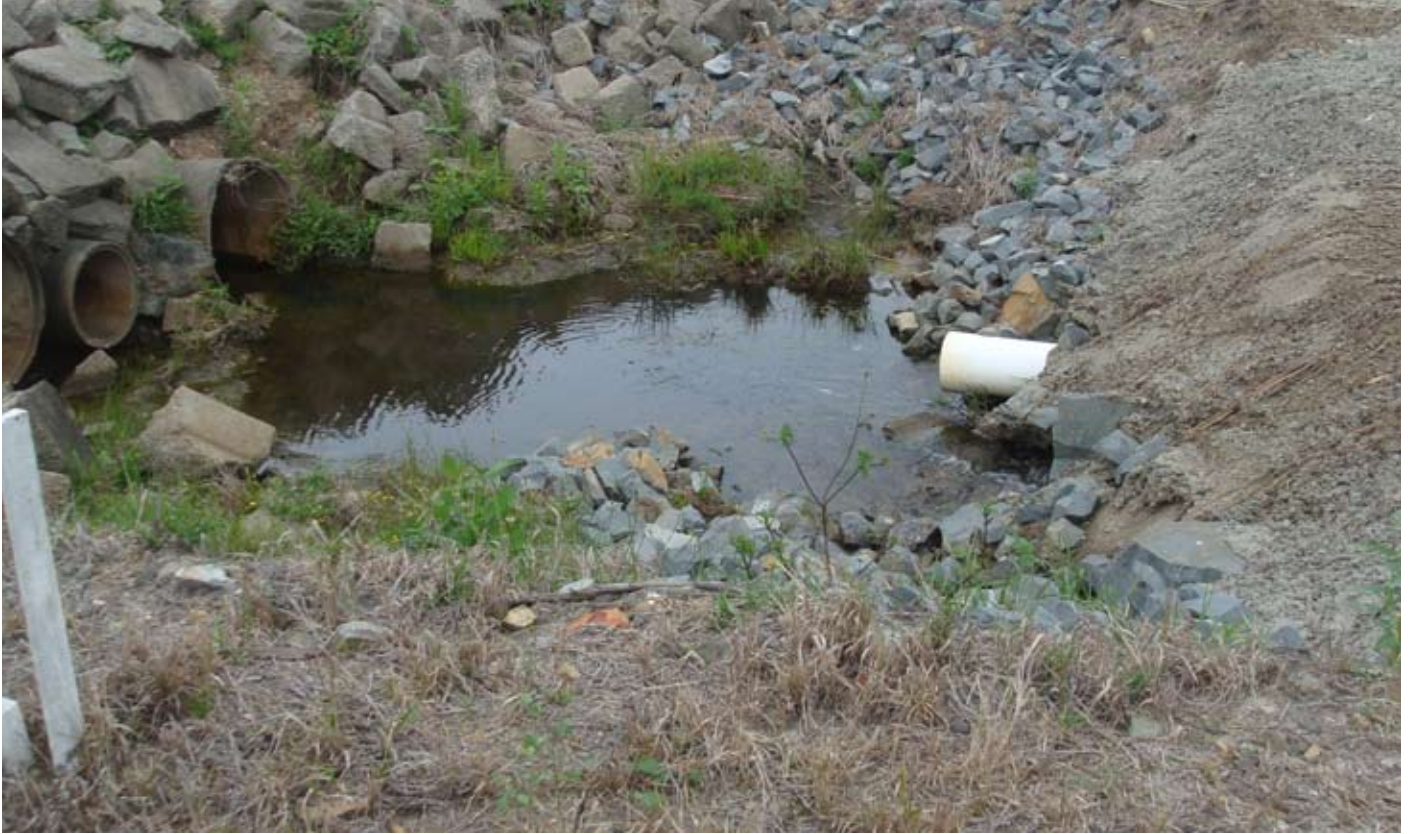
Overflow from Existing Lagoon to Duchess Gully - Temporary Outlet
