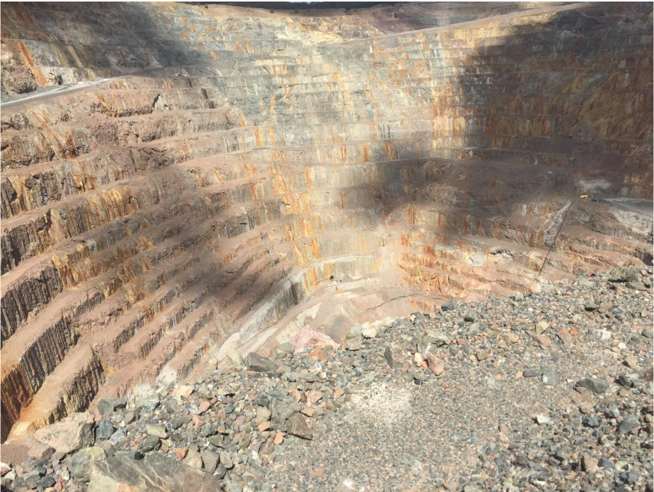
Figure 3 Photo within Cadia Hill Pit showing limited and isolated seep zones
