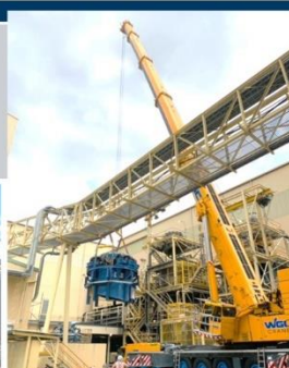
Now replacement cyclone cluster being lifted into the Con2 building by 900 T crane, during Jan 21 shutdown
