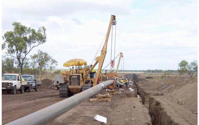
Using side-boom tractors to lower in the pipe
