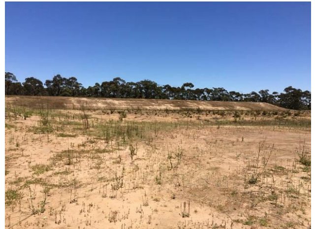
Photograph 4 – New range 50m x 140m and stopbutt
