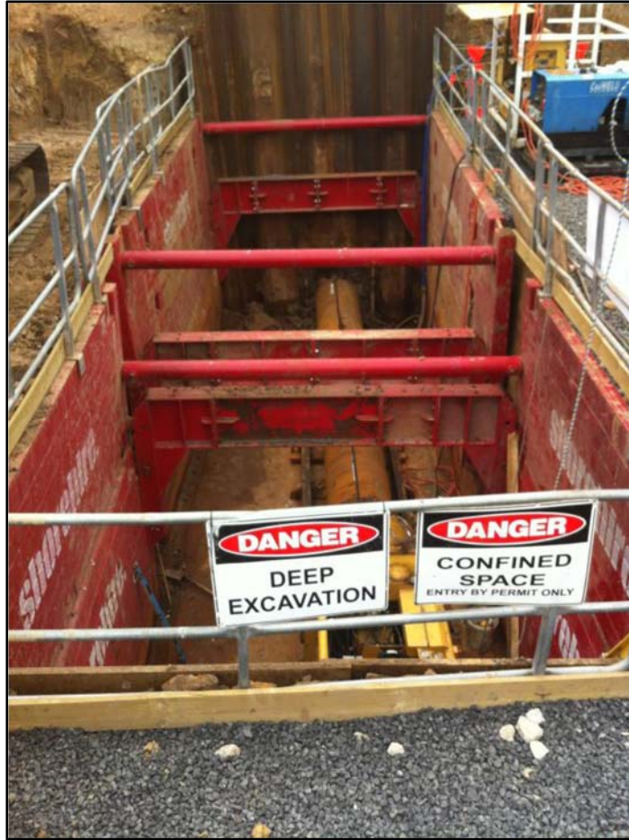
Plate 8: Installing augers and steel enveloper with auger boring machine.
