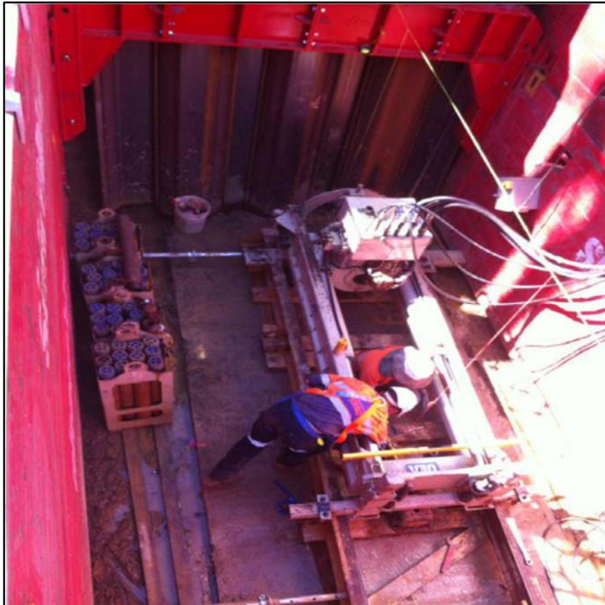
Plate 5: Setting the GBM using plumb bobs to project design line.
