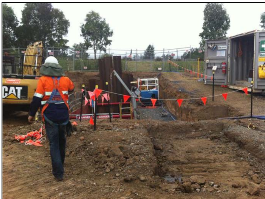
Plate 4: Launch Pit in operation.
