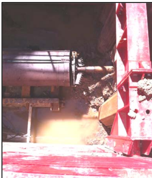
Plate 2: Lead pipe with cutting swivel head connected to pilot tubes.
