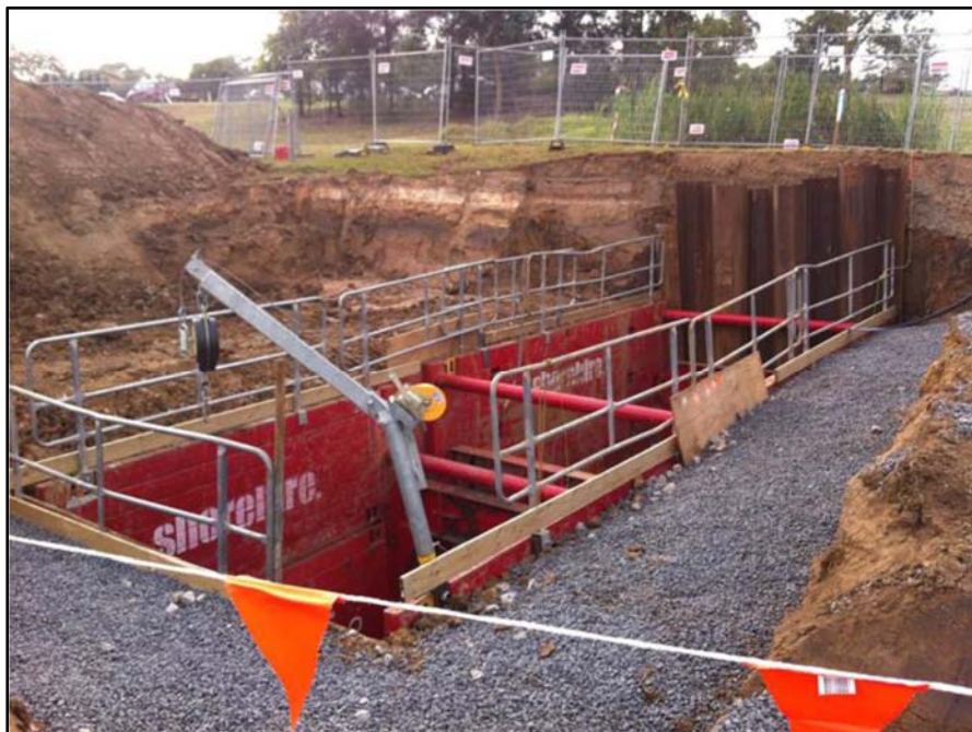
Plate 3: Launch Pit set up.
