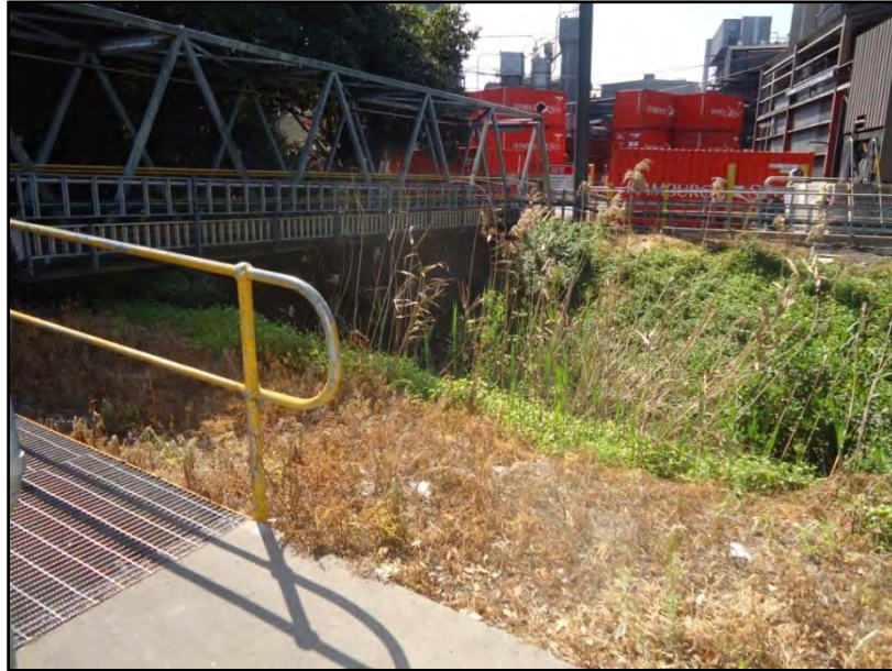
Photo No. 3: Bare soil and weeds on steep batter above Abernethy's Creek. Straw bales will be used to filter the runoff.
