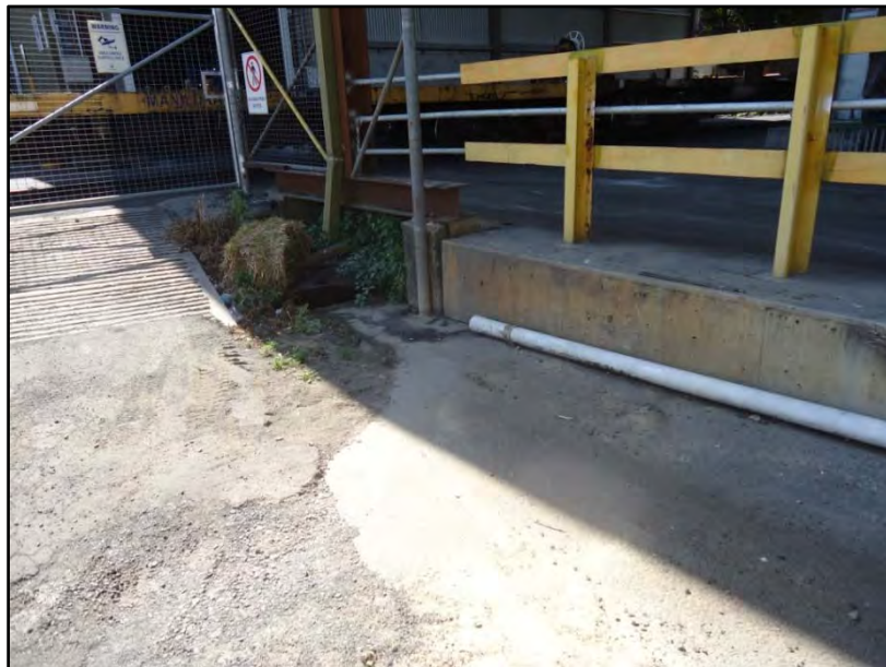
Photo No. 4: Existing straw bale serves no purpose and should be removed and replaced with a steel grate.
