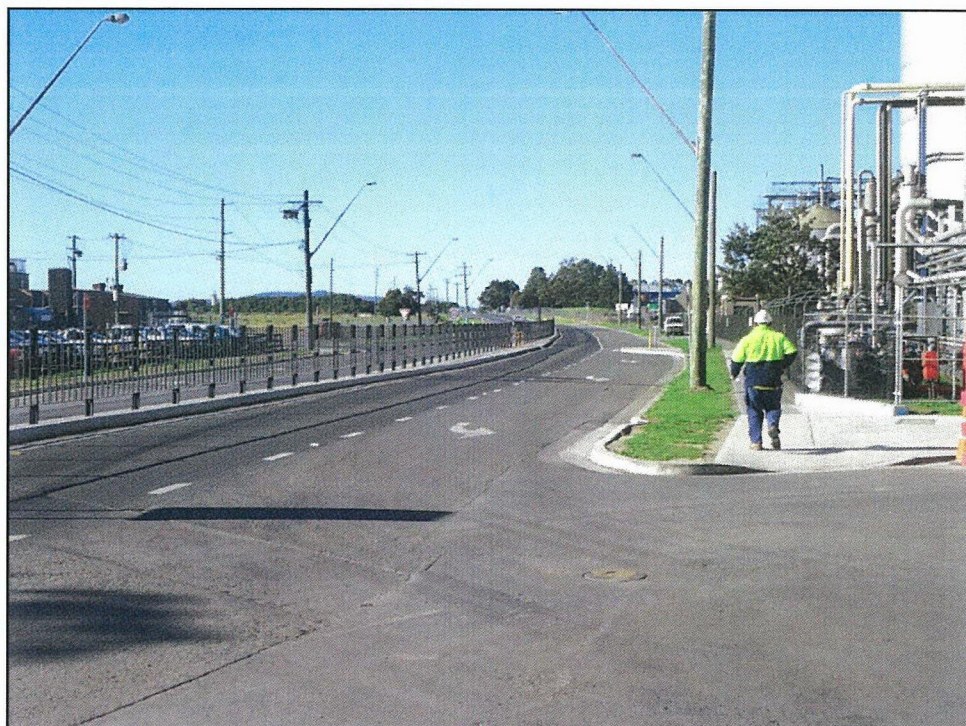
Plate 3: Channelised left turn intersection – Access Point 2.
