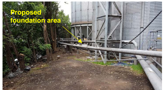
Photo 16: Looking west towards area for conveyor bucket foundations. Note potential fill within foreground of photo.
