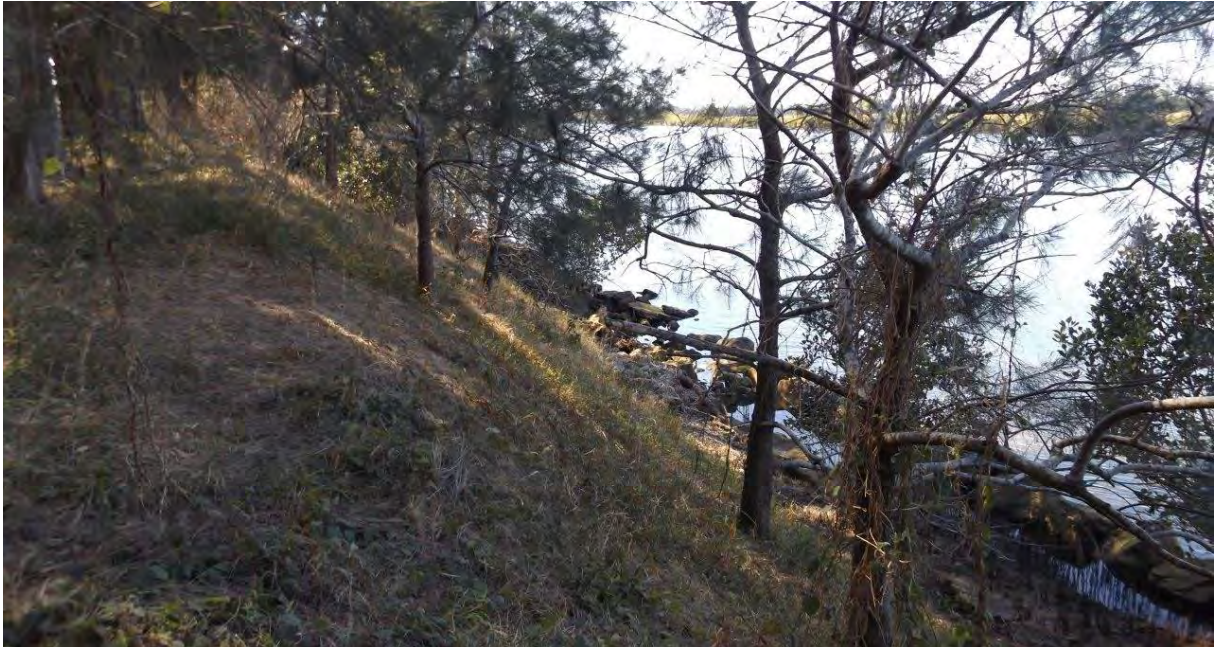
Photo 1. View looking east along riverbank showing top of bank and batter slope down to river, with large rocks placed along shoreline of river in tidal zone. Note typical vegetation in riparian zone over riverbank and along top of bank.
