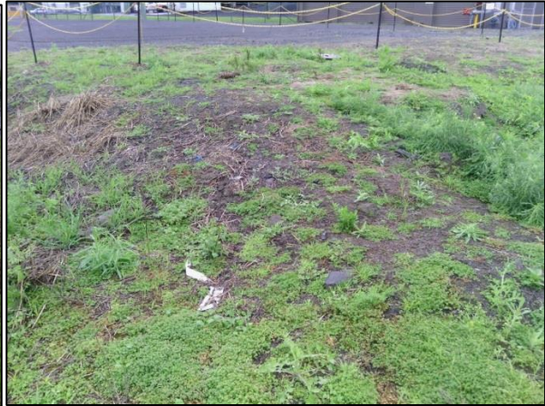
Photograph 11. Evidence of fill beneath carpark
