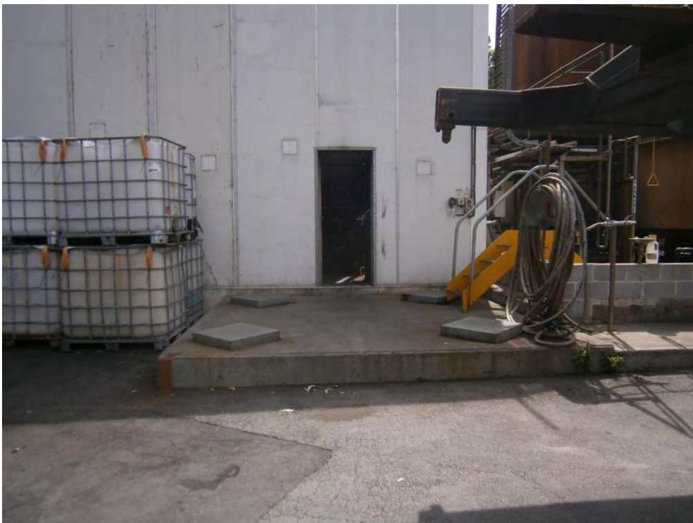
Photograph 11 – View of site for Silo from top of eastern bank of Abernethy's Creek. Concrete plinth formed for location of silo.
