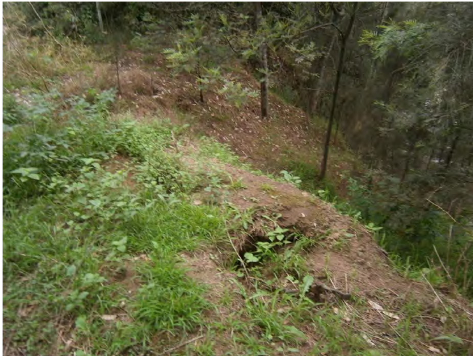
Photograph 18 – View across top of creek bank where erosion has occurred due to rabbit burrows. Undulating shape of creek bank indicates previous slumping and erosion of bank.
