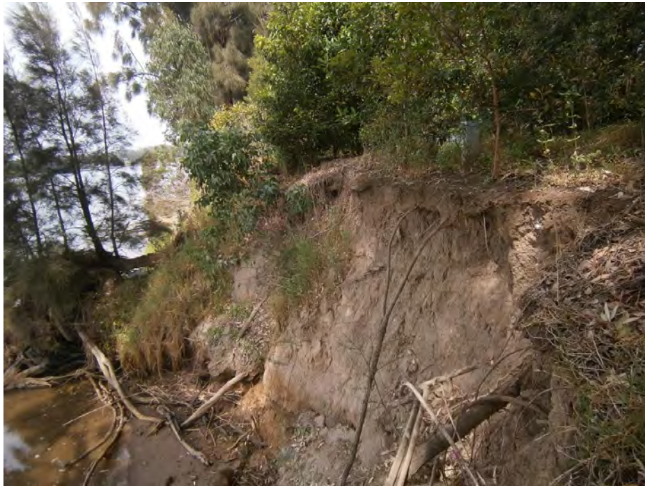
Photograph 4 – View of river bank about 25m south of biofilters showing recent erosion and collapse and edge of river at low tide.
