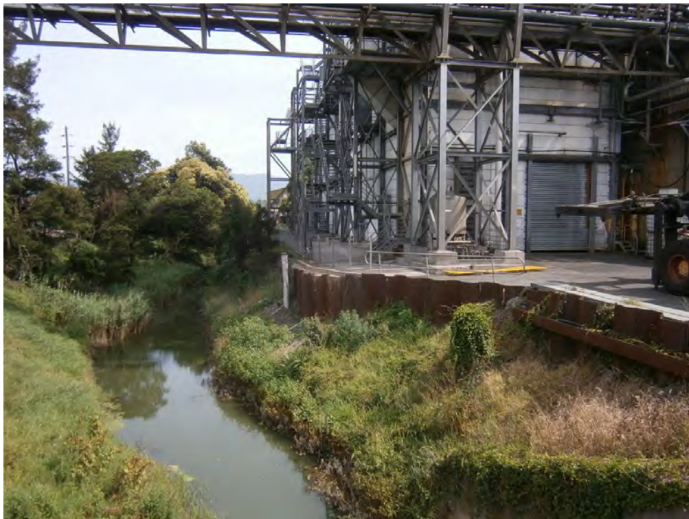
Photograph 9 – View of eastern bank of Abernethy's Creek looking north, with the site for the silo located about 5m to 10m east of the top of bank. Note sheet pile wall along top of bank supporting paved area above the bank.
