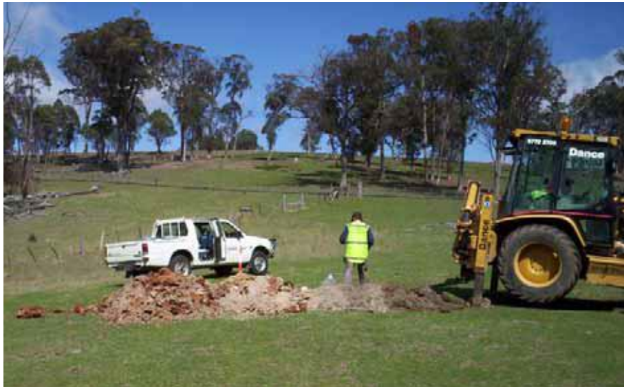
Plate 2. Pit excavation with a backhoe at Test Pit 2
