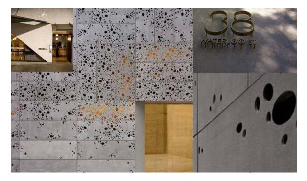
The material palette of white patterned and perforated pre cast walls (or similar) is offset by a highly articulated steel entry portal at pedestrian level. The perforations emulate the form of the iconic Illawarra flame tree and provide a playful and fluid patternation across the facade.
