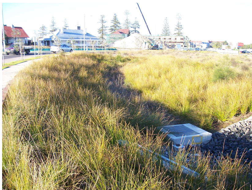
Figure 1: Example of how a vegetated swale/creek can be used for water quality control
