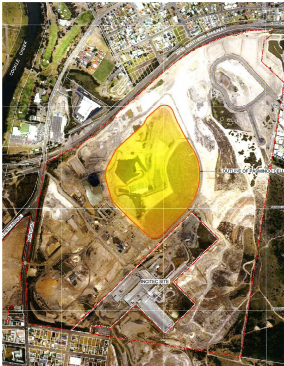
Figure 1.4 – Aerial Photo of Combined Project Cell
