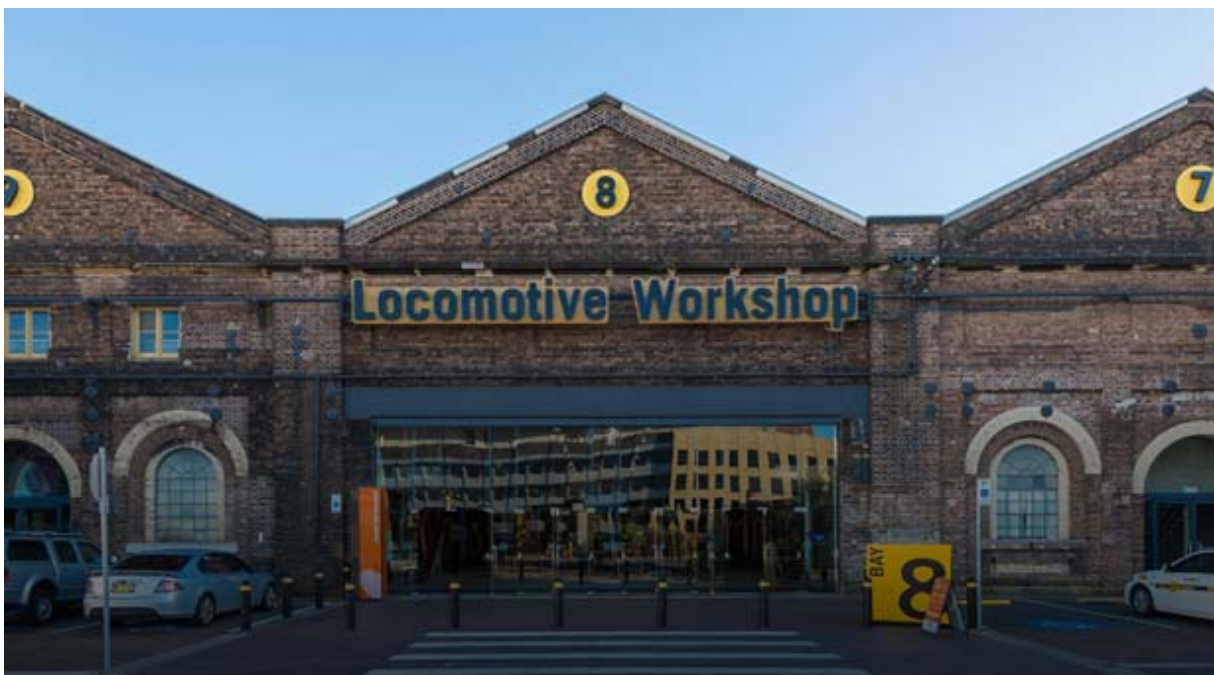
Figure 6 | Locomotive workshop (Source: Mirvac)
