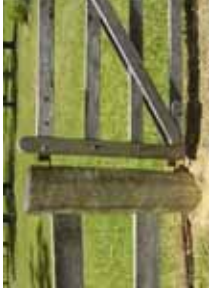
At feature locations split hwd post and rail fencing will be used in combination with bollards to permanently fence off areas of ecological sensitivity
