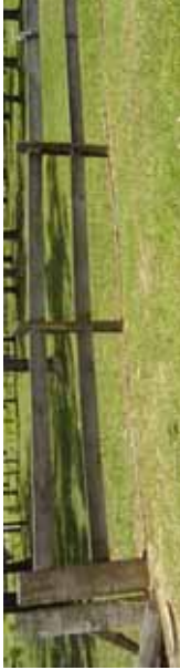
At feature locations split hwd post and rail fencing will be used in combination with bollards to permanently fence off areas of ecological sensitivity
