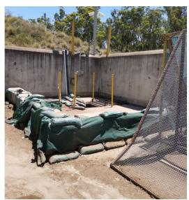
Figure 4-6: Bunded Sump Draining the Timber Waste Yard
