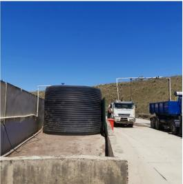
Figure 4-7: Bunded Tanks for Storing Runoff from Timber Waste Yard and Landfill Leachate
