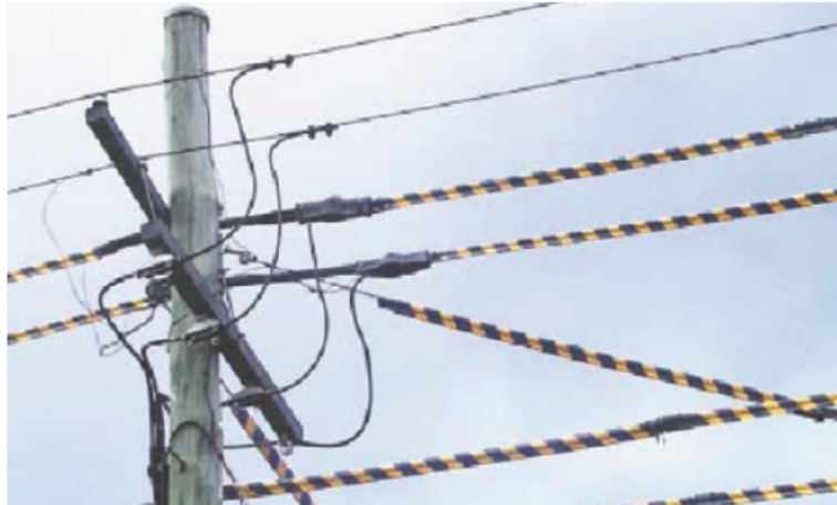
Figure 16 – Tiger tails fitted to overhead power lines
