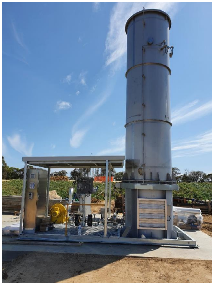
Figure 2-1: Example of the model OEF-300 flare installed for Harvey Beef, Western Australia.
