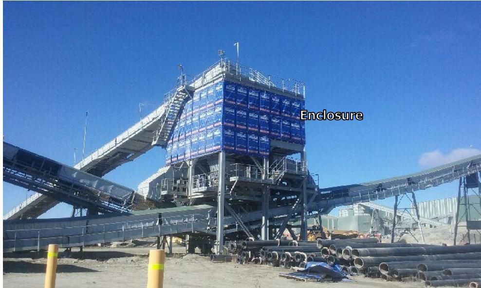
Figure 3-2 Primary Bin noise mitigation
