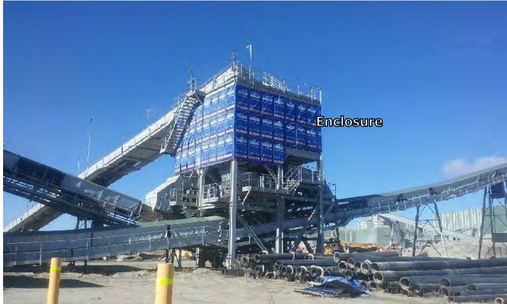
Figure 3-2 Primary Bin noise mitigation
