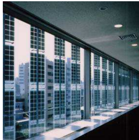
PV can be used effectively as solar shading
