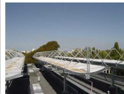
The CHAPS system at ANU. The protective coating on the mirrors is still in place and the PV section needs to be added.
