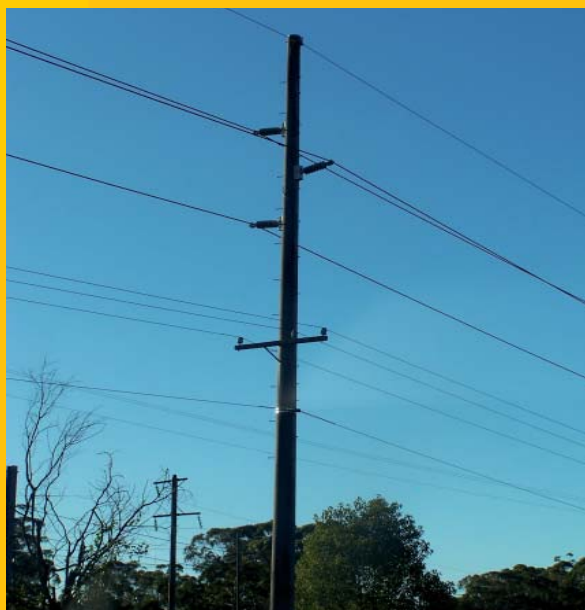
EXAMPLE OF A 33,000 VOLT LINES WITH LOWER VOLTAGE WIRES INSTALLED BELOW
