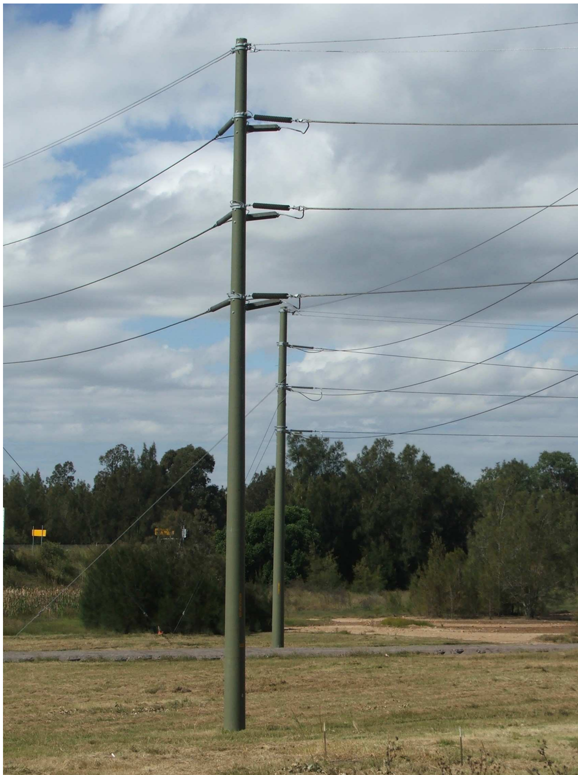
Pic 2 - Typical strain construction method
