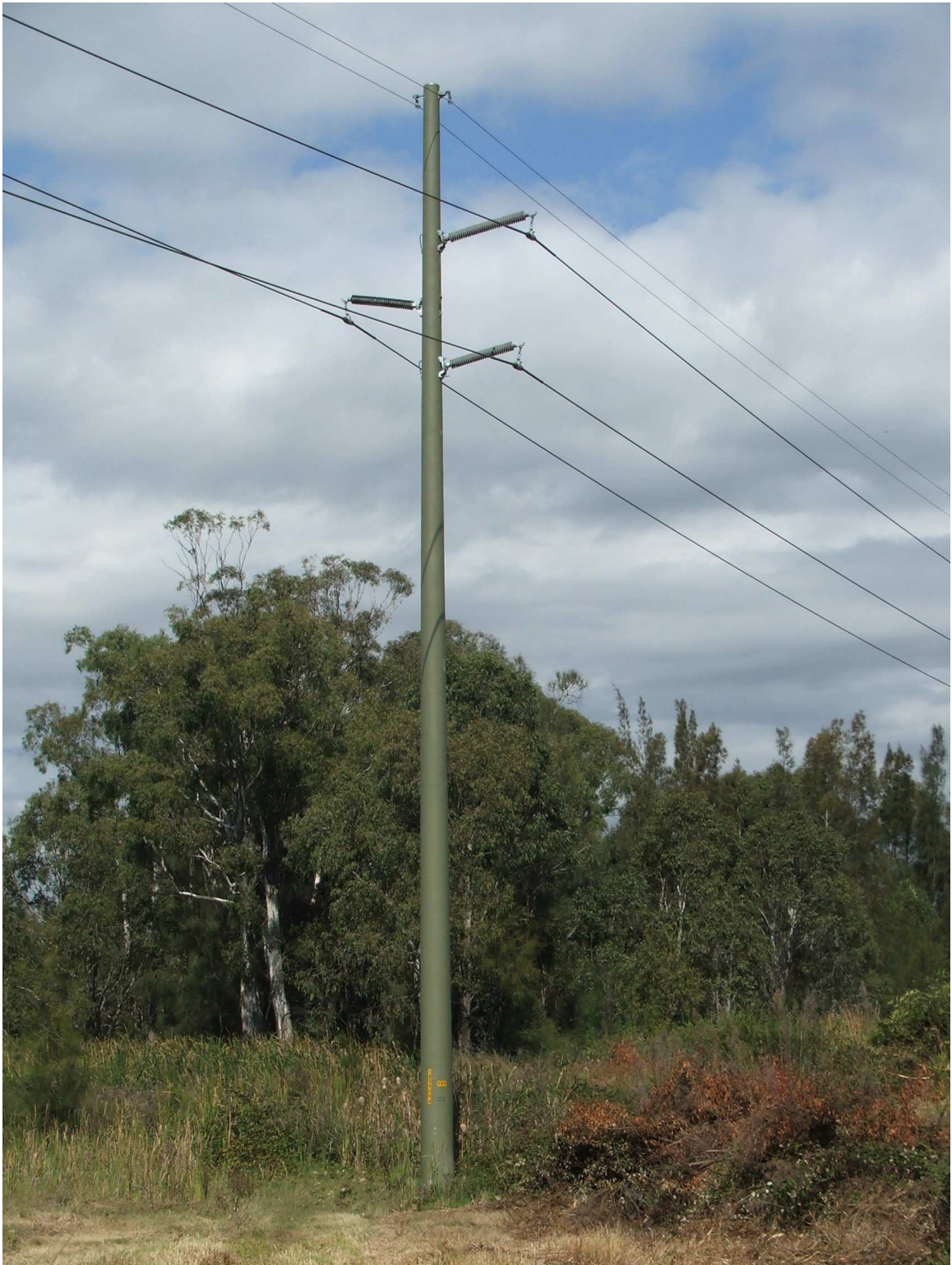
PIC 1 - Typical intermediate construction method
