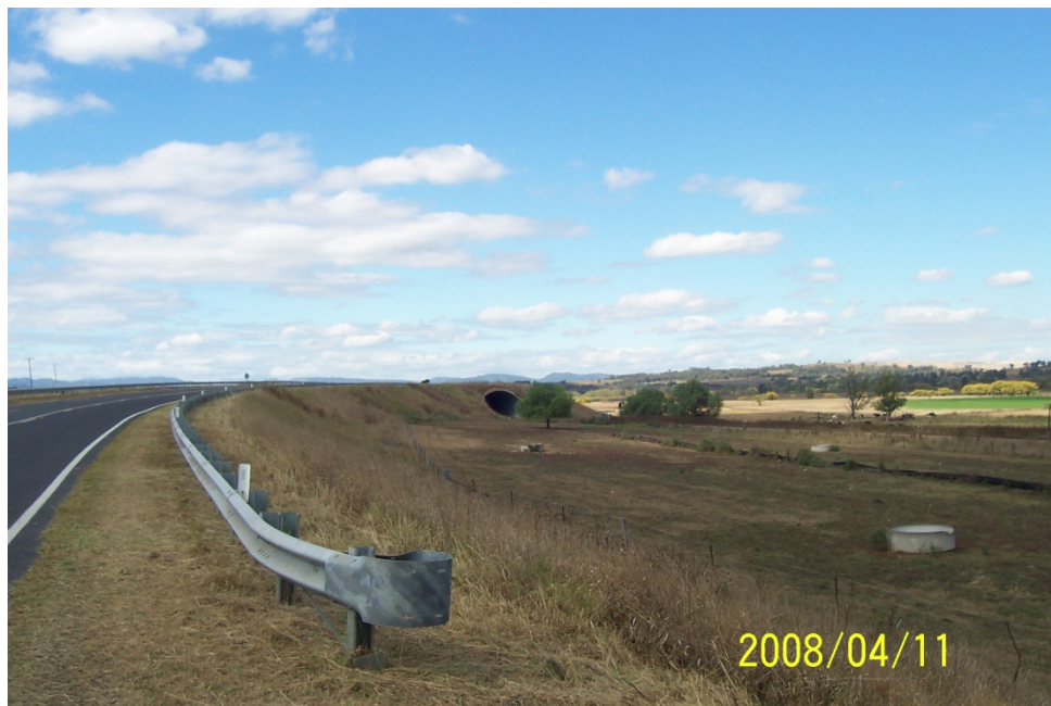
Photo 5.6 Bengala Mine Culvert Bengala Rd. Potential culvert strengthening required.
