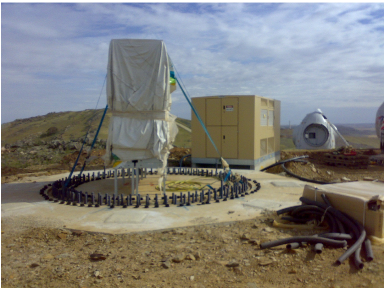
Figure 3.3 Typical Concrete Wind Turbine Foundation
