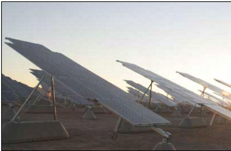
Figure 2.7 – Solar PV Single Axis Power Tracker Supporting Structure (Example)
