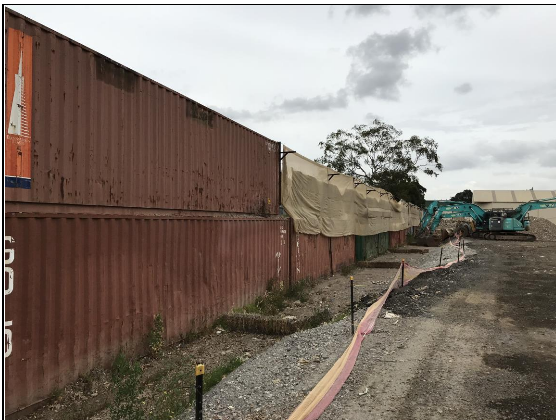
Plate 4 – Containers used to attenuate noise emissions from processing activities
