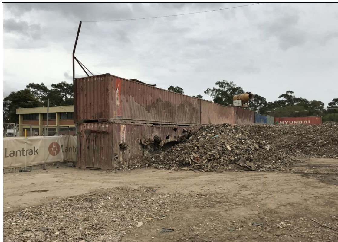
Plate 4 – Containers used to attenuate noise emissions from processing activities
