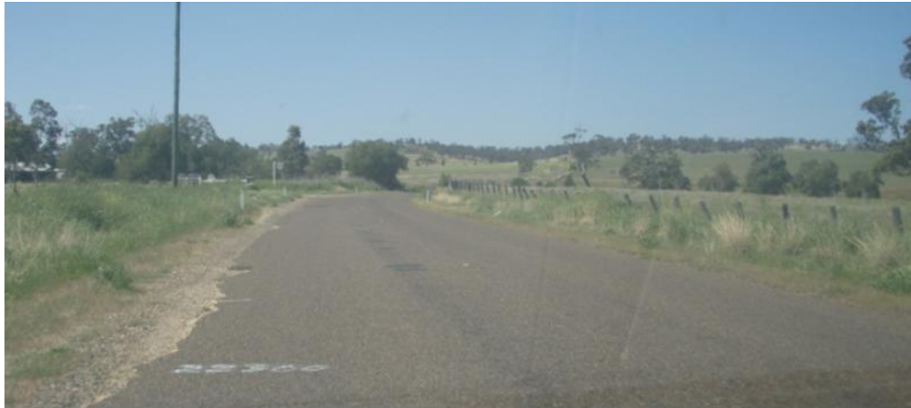
Figure 2-5 Degradation of edge of seal on Wybong Road, east of Mangoola Road
