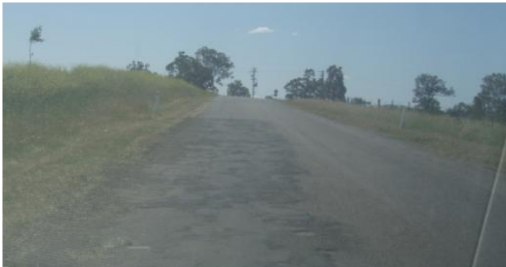
Figure 2-6 Excessive patching on Wybong Road
