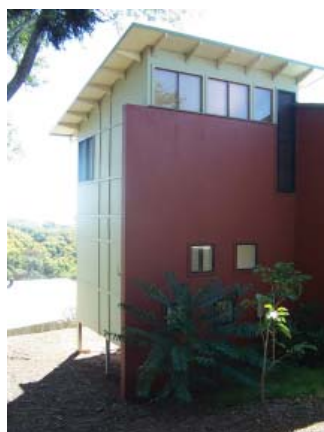
Site responsive methods of construction with lightframe buildings and suspended floors
