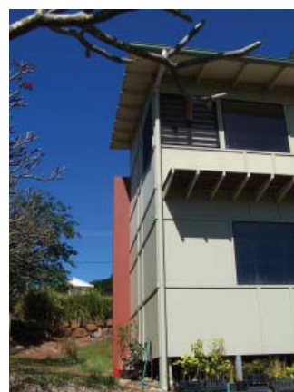
Site responsive methods of construction with lightframe buildings and suspended floors
