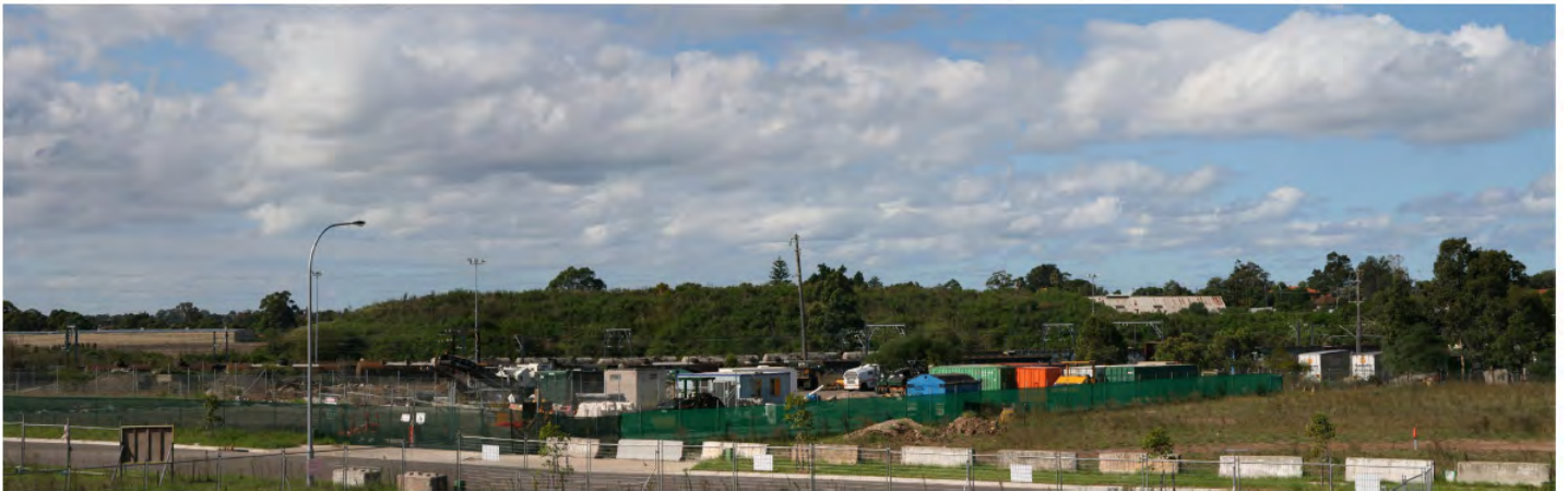
Figure 3.3: Existing View from Wentworth Street facing east
