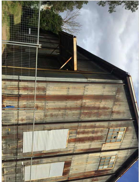
1. VIEW FROM COSGROVE ROAD ENTRY
