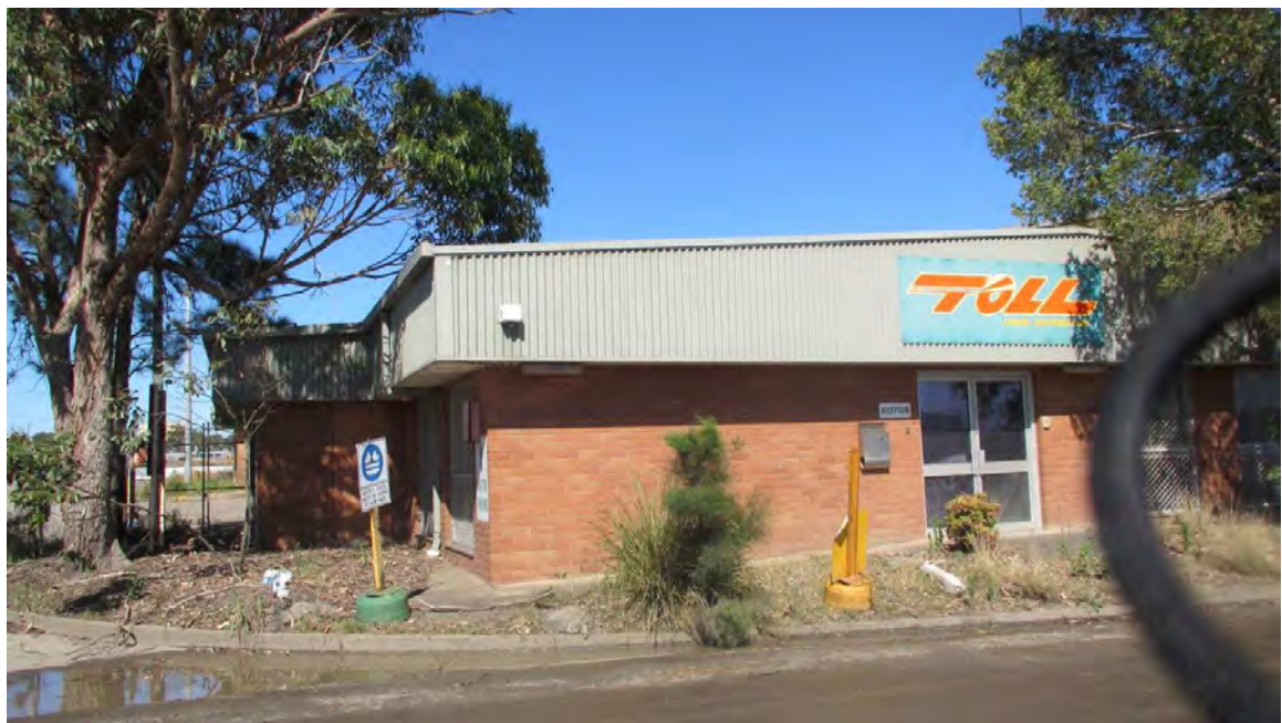
Photo 8: Former Toll office building, looking west
