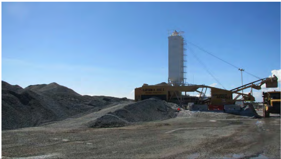
Photo 7: Pugmull and DGB stockpile, looking north
