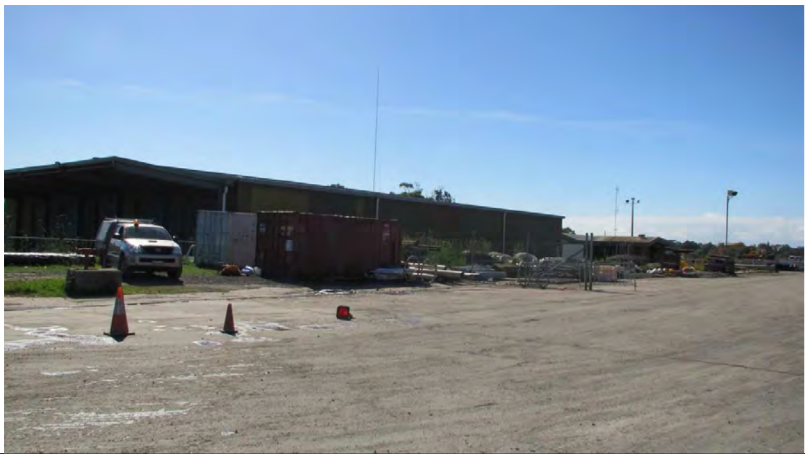
Photo 3:Construction material storage area in the centre of the site, looking south-east
