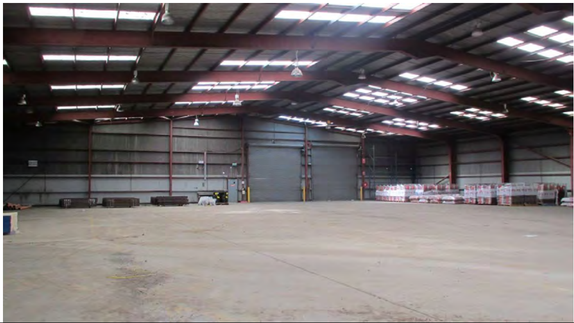
Photo 1: Inside the former Toll building
