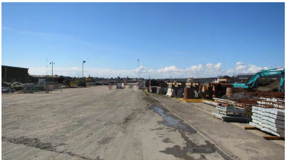
Photo 2: Construction material storage and parking area along western site boundary, looking south
