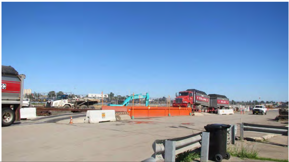
Photo 5: Weighbridge located in the western portion of the site, looking west
