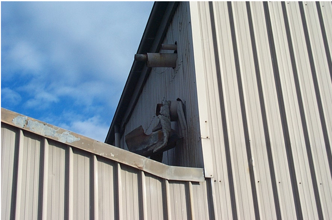
Figure 5. Exposed insulation from lagged pipes (northern end of Building 5)
