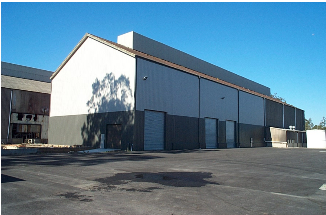
Figure 4. Workshop After New Cladding and PVA-coated Asbestos Cement Sheets
