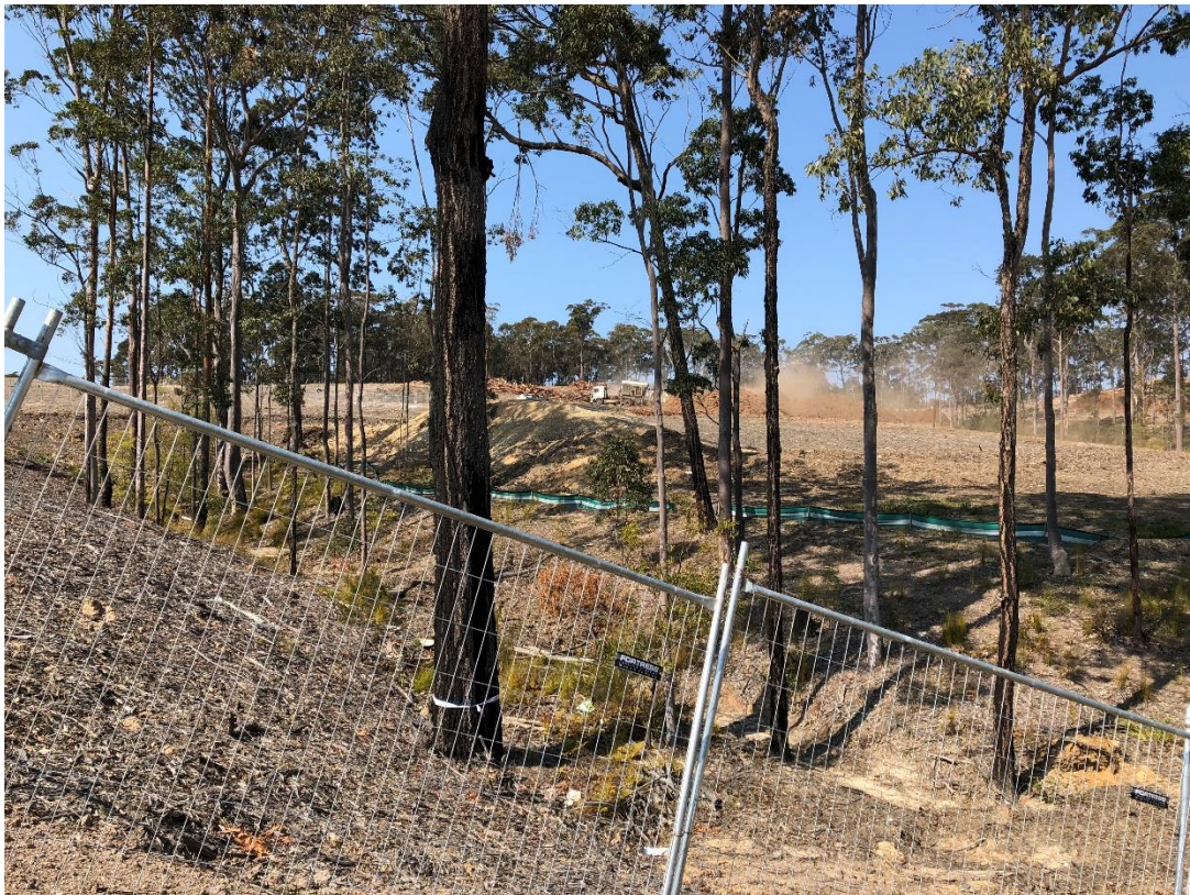
Figure 4.1: Subject site - view upslope along drainage line
