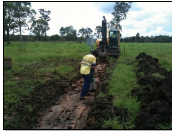
2. Trench re-filled and compacted in layers.
