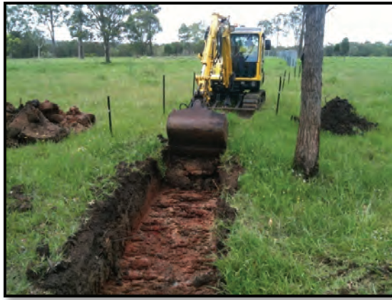
1. Excavator removes soil down to the base of cracking.
