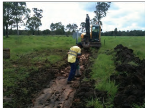
2. Trench re-filled and compacted in layers.
