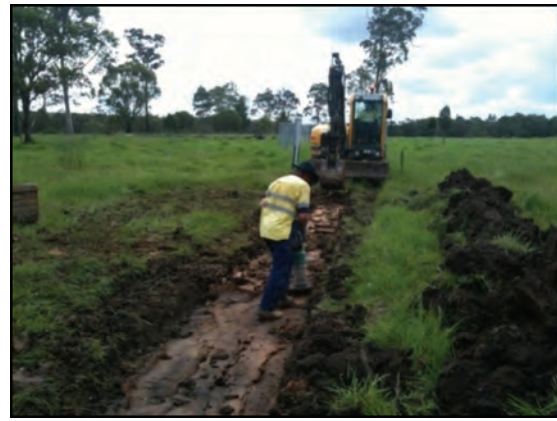
2. Trench re-filled and compacted in layers.
