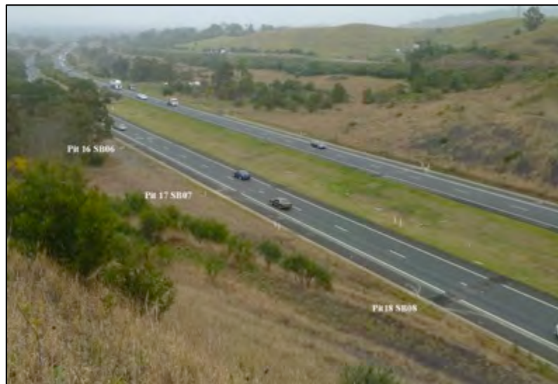
This section of the Hume Highway has been subsided and successfully rehabilitated
