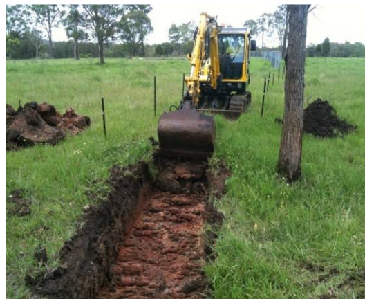
Plate 6 – Example of Subsidence Remediation
