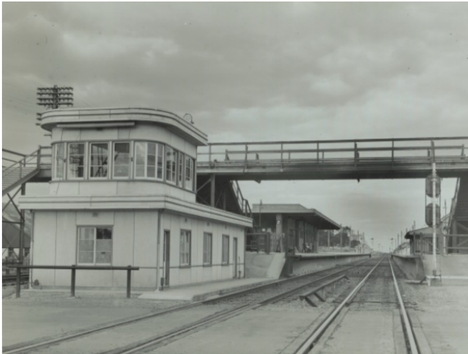
Figure 17. St Marys Station, 1945. This photograph illustrates the non-standard signal box, a precursor to post-war S-type signal boxes. 35
