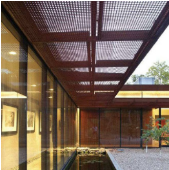
CAN-01 Steel Framed Cantilevered Glazed Awning with integrated frit Colour: Black Framing/Bronze Frit
