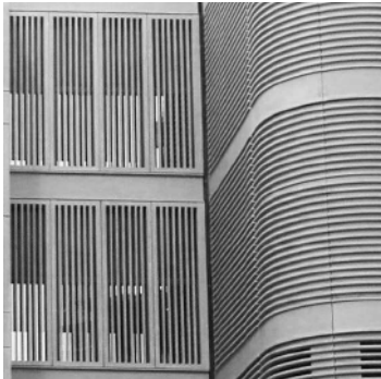
CON-01 Glass Reinforced Concrete Blades (GRC) Colour: Acid Wash with Micro Aggregate Finish
